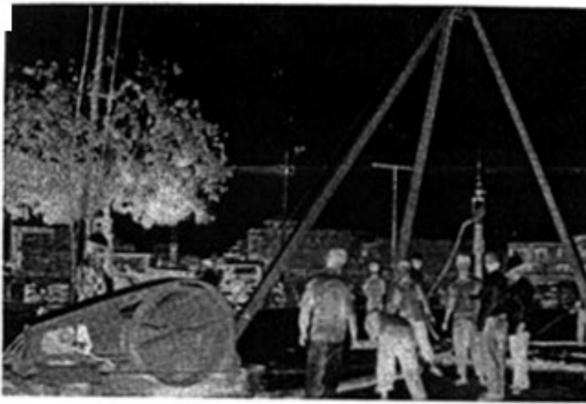
Fig. 4 : Photographs Showing Bored Piling by DMC Method in Progress at JLN Marg, Jaipur.
