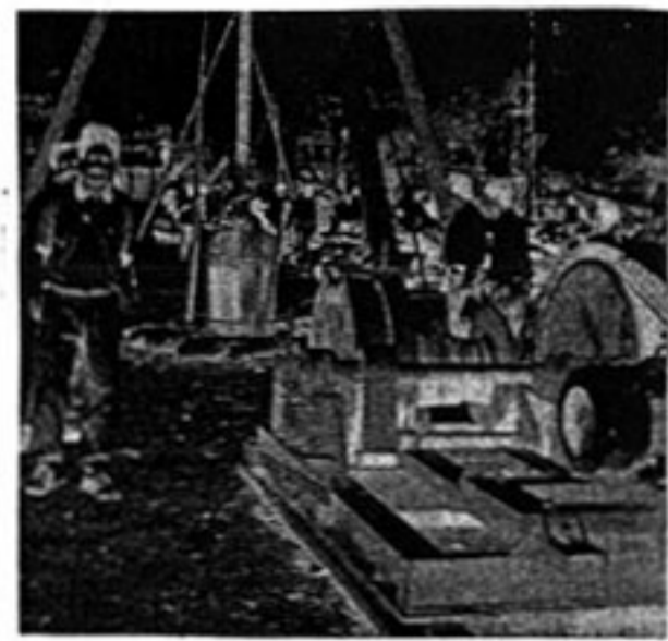
Fig. 4 : Photographs Showing Bored Piling by DMC Method in Progress at JLN Marg, Jaipur.
