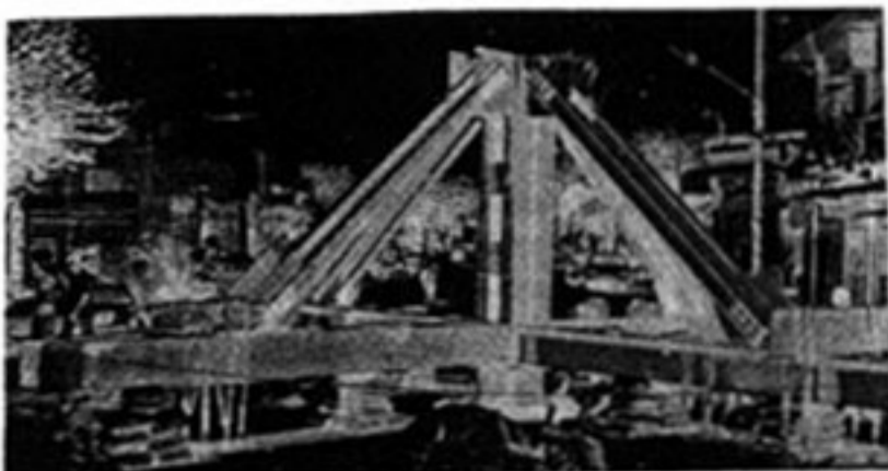
Fig. 5 : Load Frame for Pile Load Test
